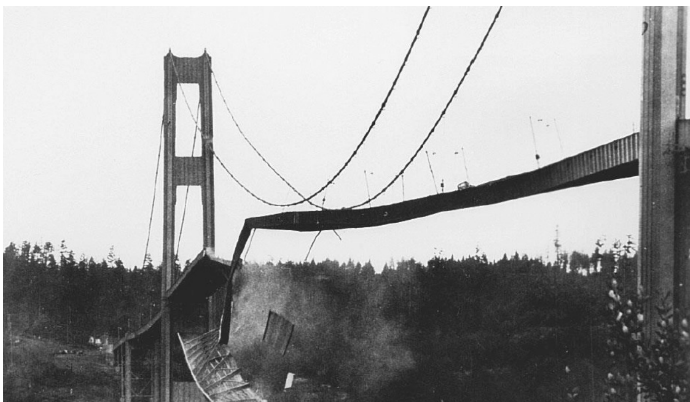
Tacoma Narrows Bridge 1940 Wind induced vibrations
